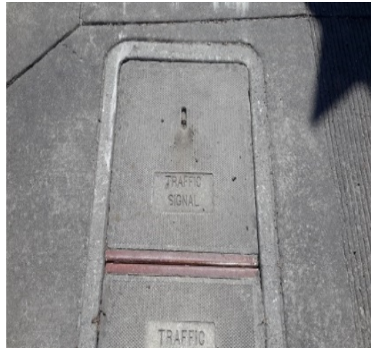
Traffic Signal Box Lid
