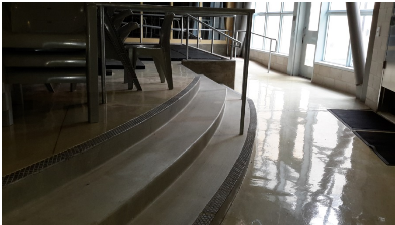
Detention Unit- Steps and Ramp from Dining/Activity Area to Cells, Showers and Outside Exercise Yard
