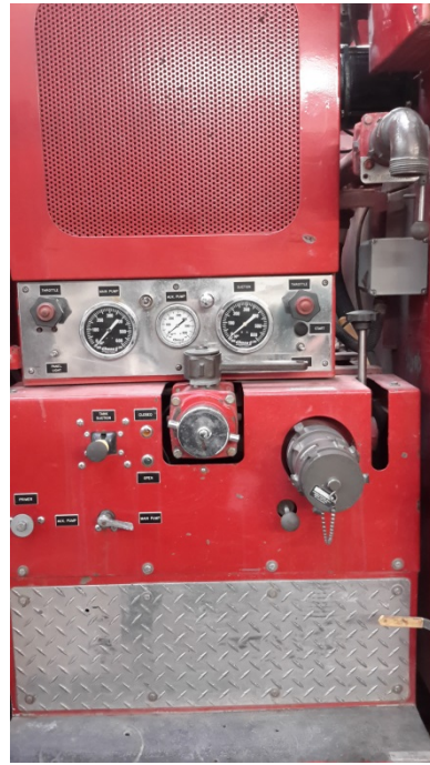
Fire Truck- Water Pressure Guages
