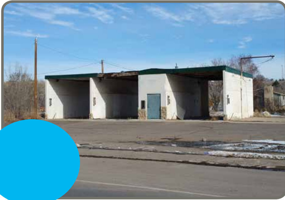
Former Gas Station
